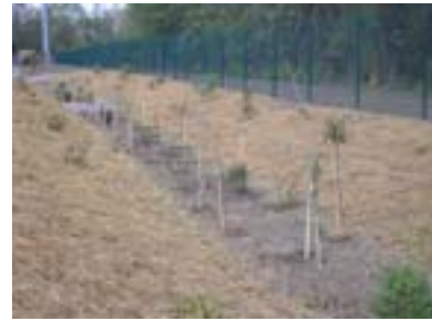
Example of Bioswale Planting
