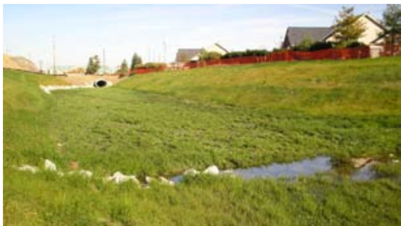
Application of over-wide channel technique. Source: EMH&T
