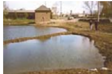
Example of Chemical and Biological Treatment Tanners Lake alum injection facility — Oakdale, MN
