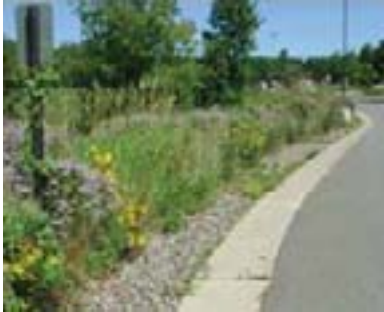
Example of Infiltration Practices Infiltration trench, Lino Lakes City Hall — Link Lakes, MN
