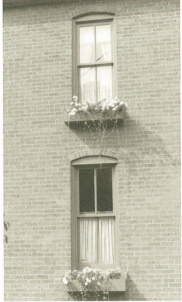
[Photo 21] Appropriately designed wood replacement windows.
