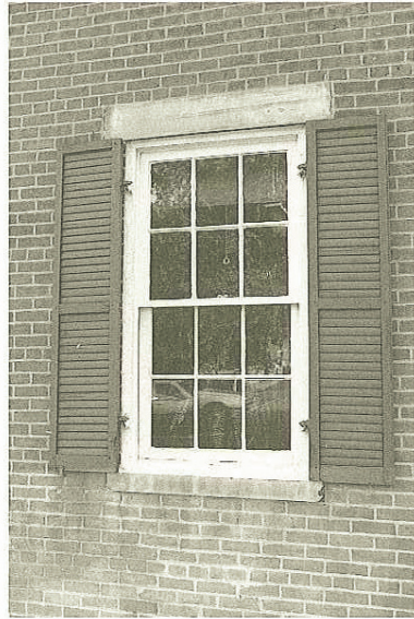
[Photo 8] The stone lintel and sill of this window have never been painted.
