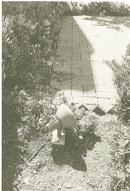
[Photos 63 and 64] Contemporary site lighting fixtures can be concealed in landscaping or placed unobtrusively under a building's eaves.
