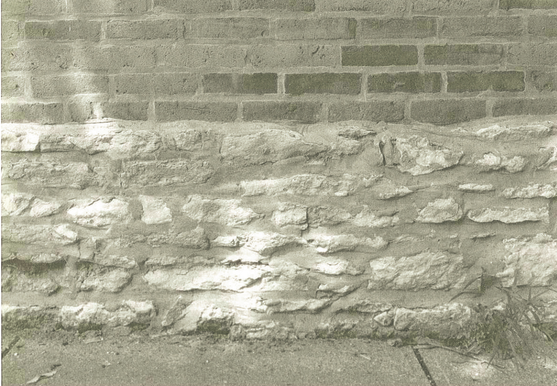
[Photo 3] A coursed rubble limestone foundation.
