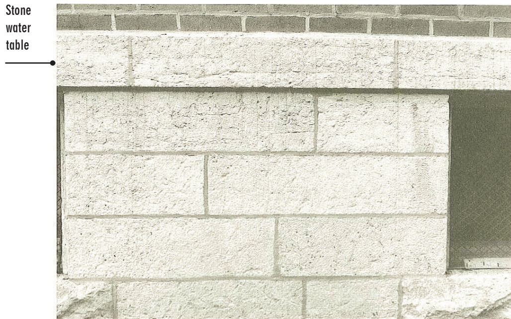
[Photo 1] A smooth-faced limestone foundation with a stone water table.
