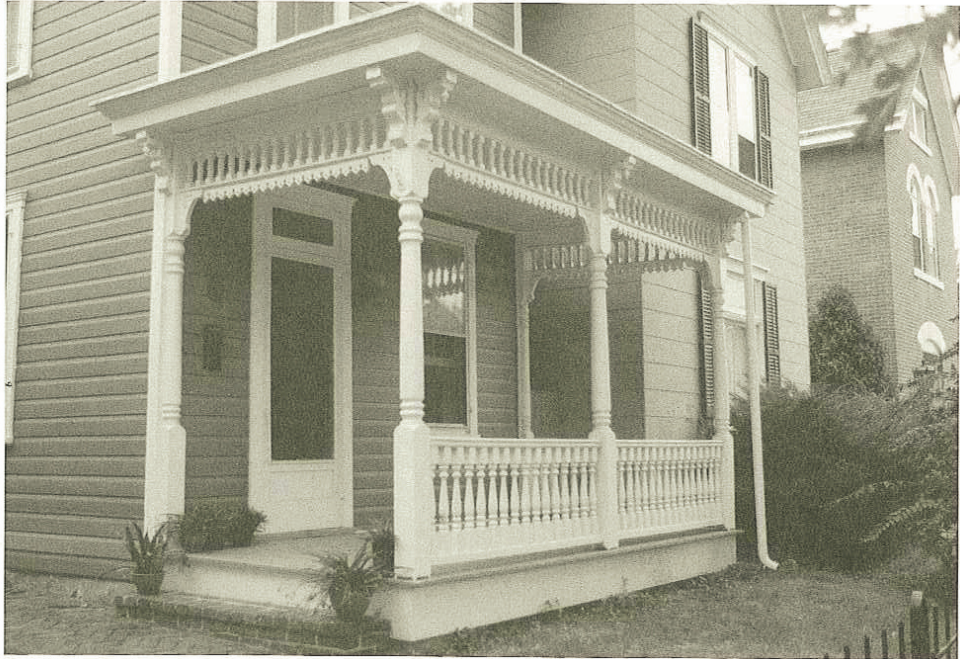
[Photo 28] A well-done repair job on an original porch.
