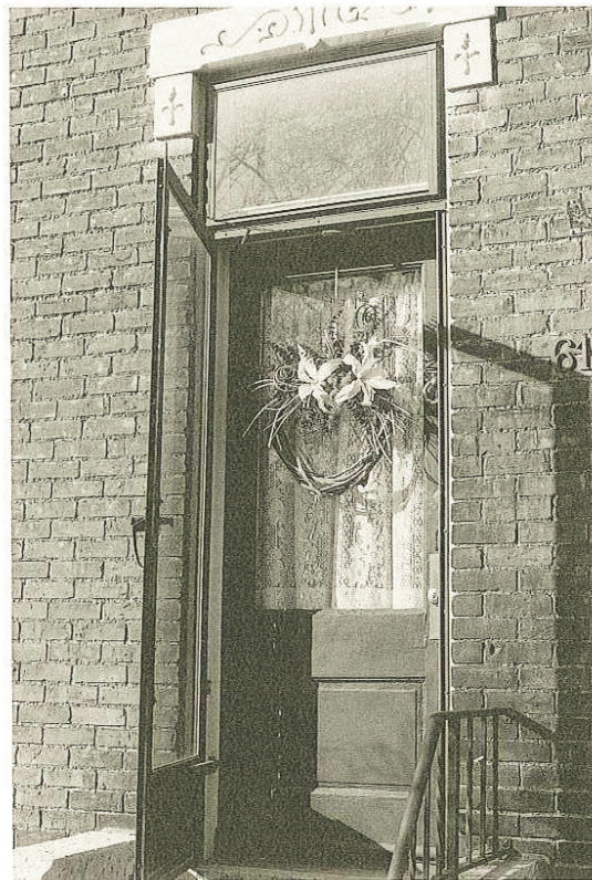
[Photo 19] A typical late 19th-century front door with a large window. Note how the transom has its own fixed-in-place storm window.
