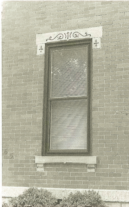
[Photo 32] Highly decorative stone lintels are a feature of many German Village houses.
