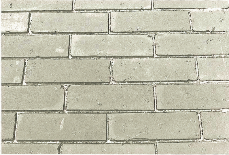
[Photo 6] Early 20th-century masonry with very narrow mortar joints.
