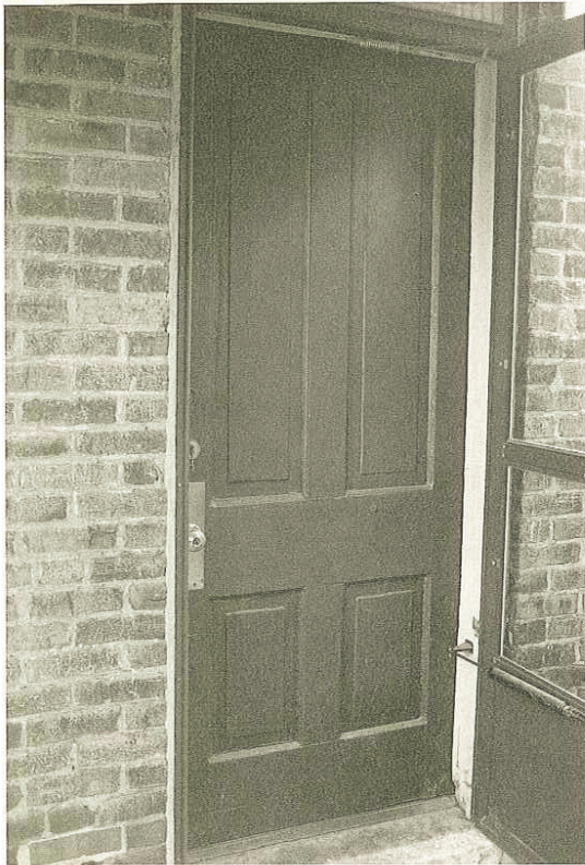
[Photo 18] A four-panel door typically found on early story-and-a-half cottages and often used on later Italianate buildings as well.
