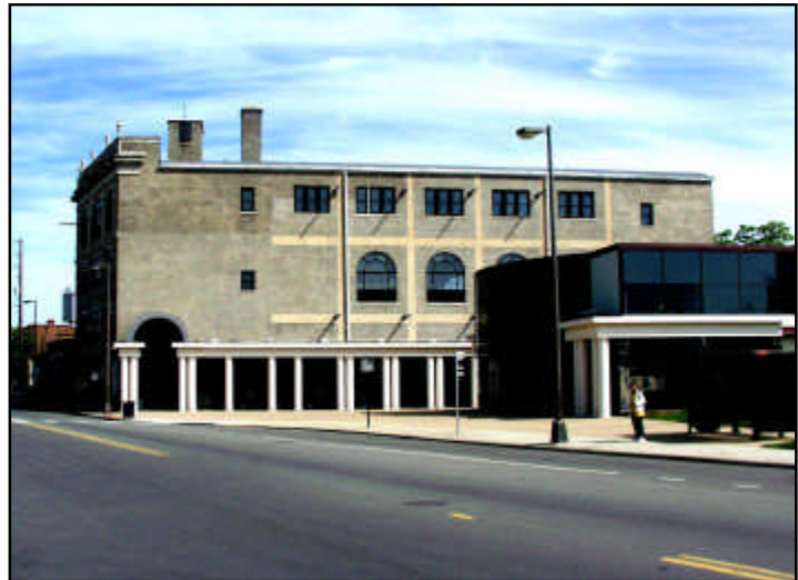
The King Arts Complex -- Mount Vernon Avenue just west of Monroe Avenue.
