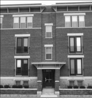
An example of contemporary architecture utilizing traditional features such as brick, vertical windows, water table, and lintels (Renaissance Condominiums in downtown Columbus). Sixty-three percent of the parking is provided by parking garages underneath the apartment structure, entered off of a rear drive.
