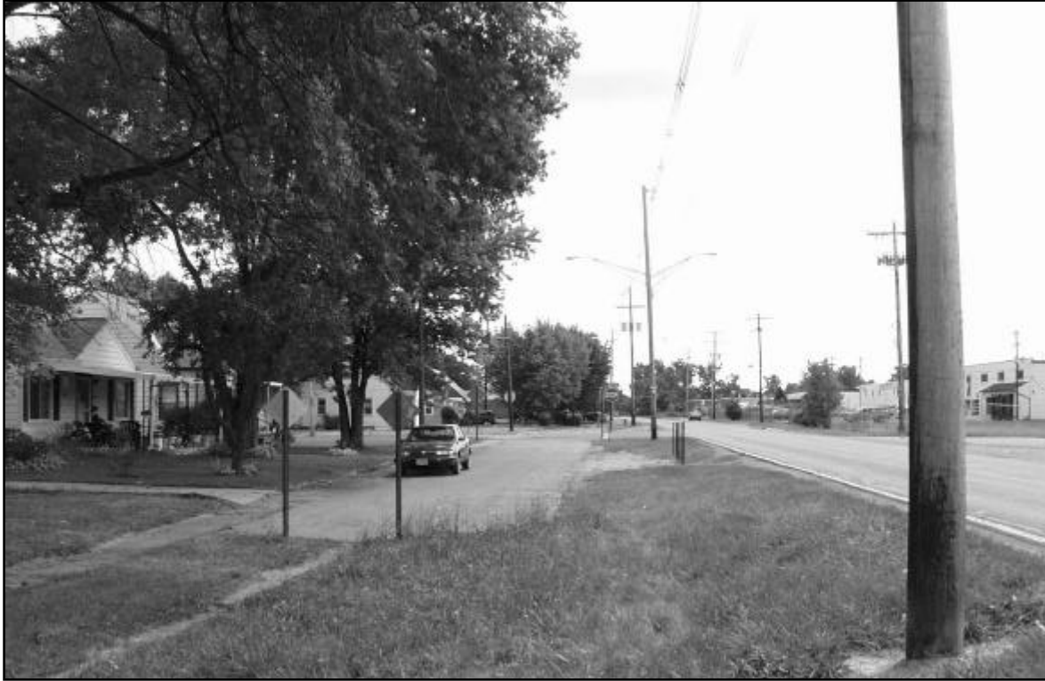
Open ditches along Woodland Avenue.
