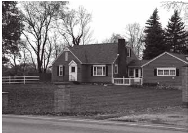
Residential building on Brown Road
