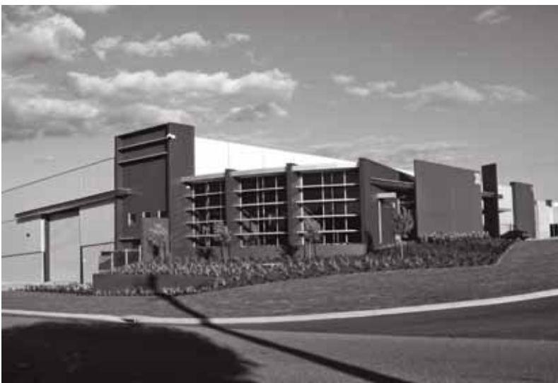
Example of industrial building with architectural character
