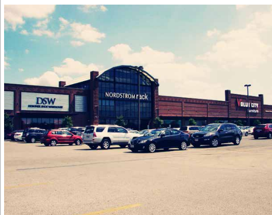
The primary parking lot within the Sun Center is hidden behind outlot development on Sawmill Road and SR 161
