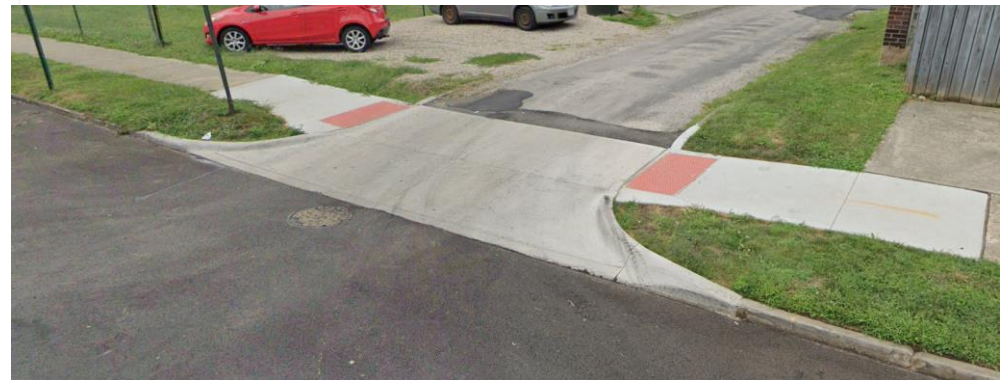
Blended transition at a raised PAR
