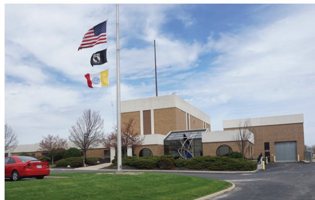
Parsons Avenue Water Treatment Plant
