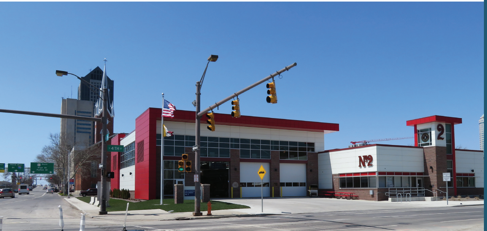
Columbus Fire Station #2
