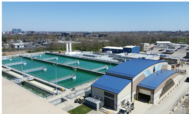
Dublin Road Water Treatment Plant
