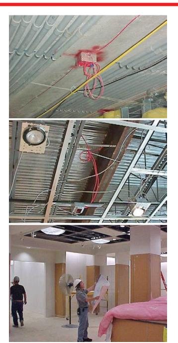
B. At the stage that the contractor has installed the alarm device boxes and wiring in the rough ceiling (e.g. smoke alarms, heat detectors, etc.) it will be necessary that these installations be inspected by the Electrical Inspector.
