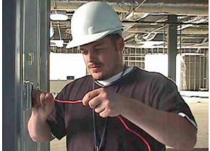
A. At the stage the contractor has installed the alarm device boxes and wiring in the rough walls (e.g. pull stations, horns, strobes, etc.) it will be necessary that these installations be inspected by the Electrical Inspector.
