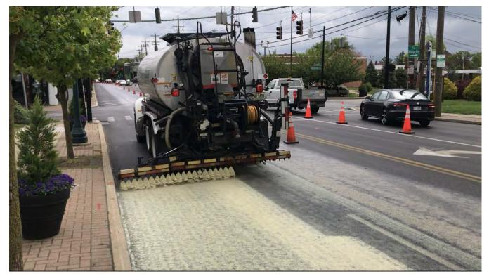
**A.R.A.-1** Ti<sup>®</sup> is a specialized version of a Maltene Replacement Technology (MRT) product enhanced to impart both the regenerative properties of a maltene rejuvenator and the beneficial sustainability and environmental properties of imbedded photocatalytic grade Titanium Dioxide (TiO<sub>2</sub>).
