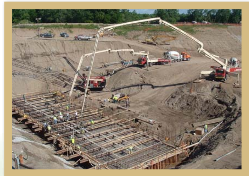
Southerly Wastewater Treatment Plant, New Headworks
