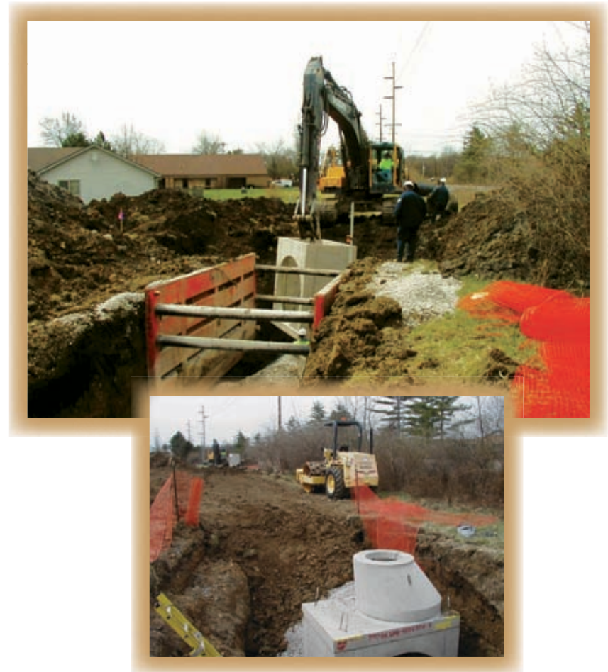
Briggs Road Storm Sewer Installation
