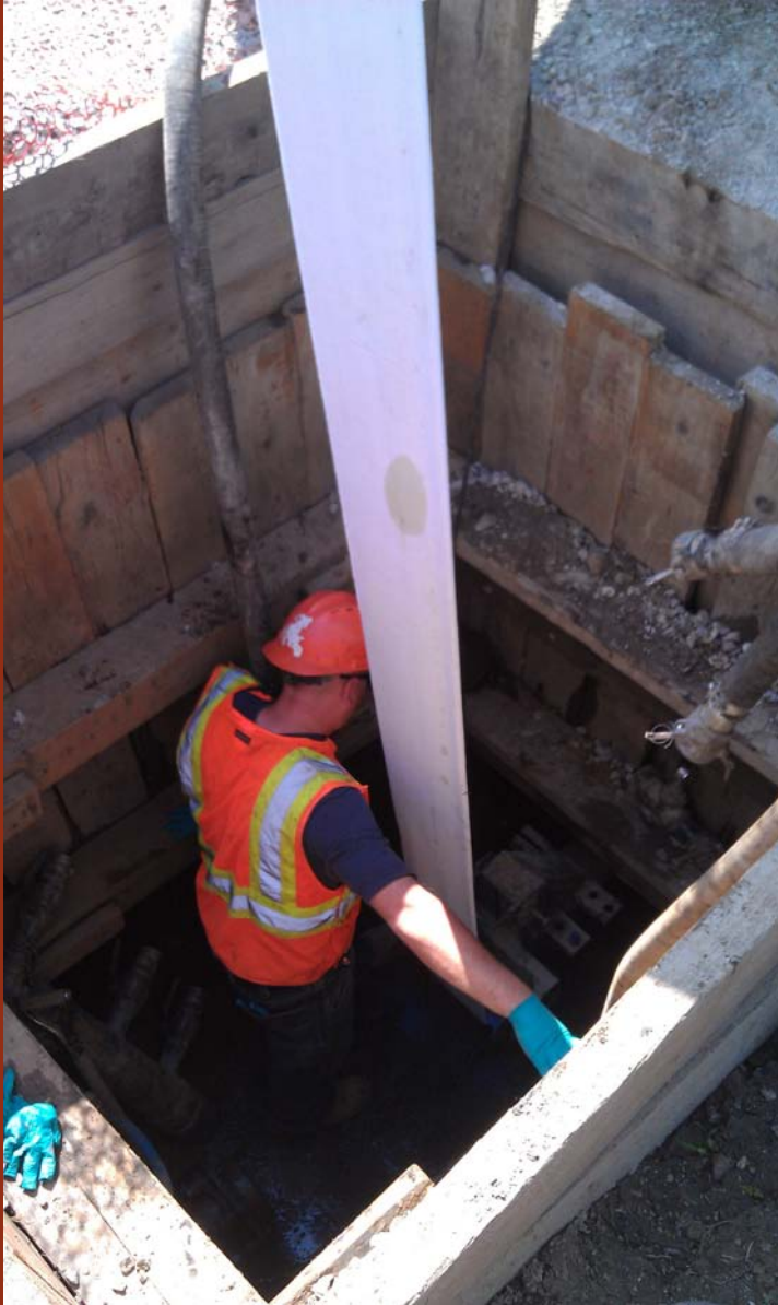
Waterline rehabilitation process
