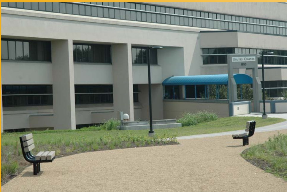
Columbus Utilities Complex, 910 Dublin Road
