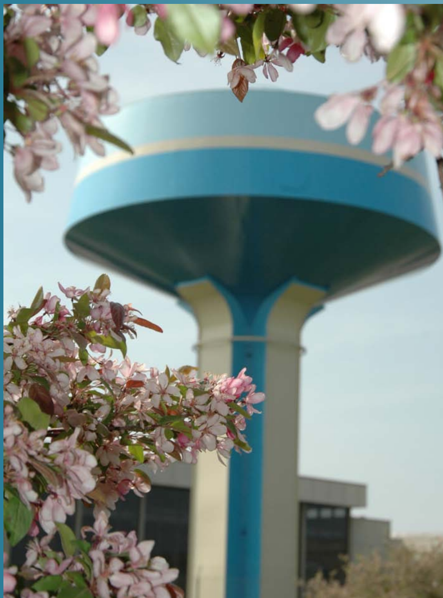
Dublin Road Water Tank
