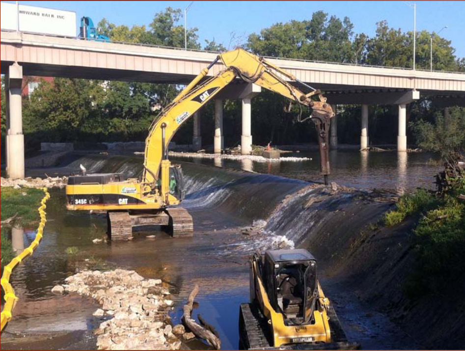
5th Avenue Dam demolition
