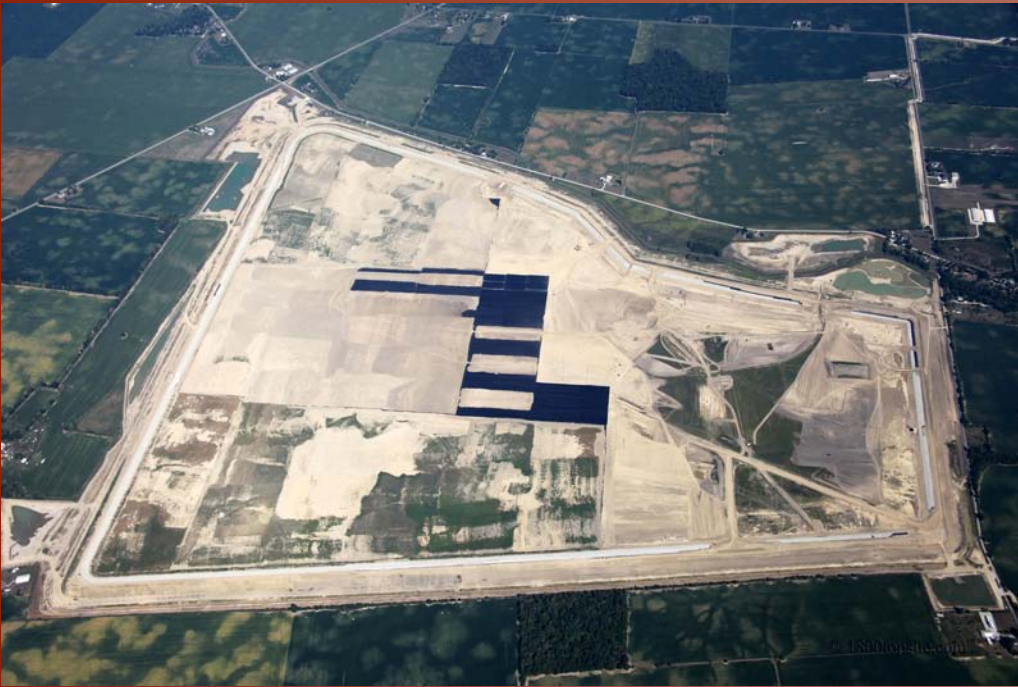
Aerial view of Upground Reservoir progress as of August 2012
