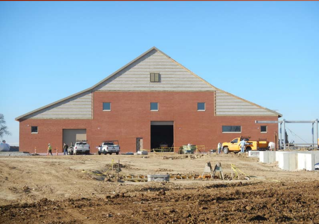
Pump station for Upground Reservoir construction underway
