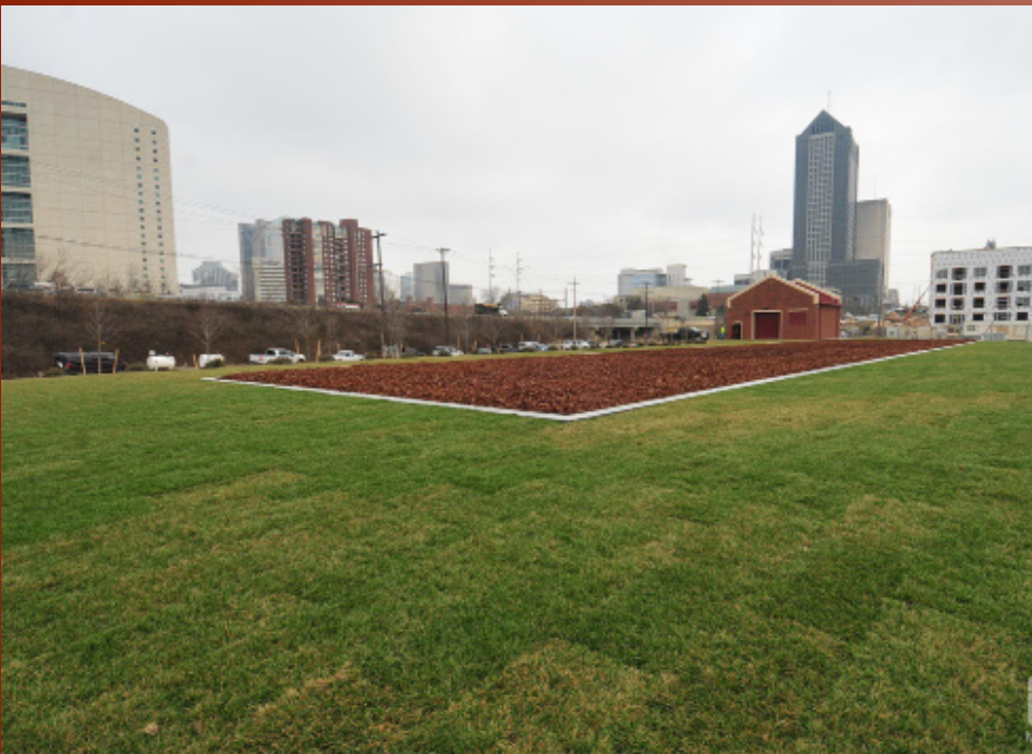
OARS shaft and biofilter
