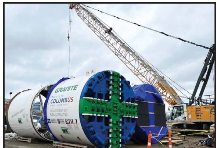
Tunnel boring machine for Lower Olentangy Tunnel at Gowdy Field
