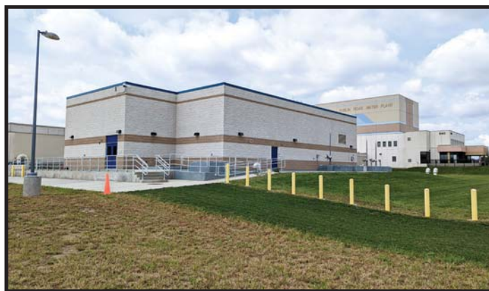
The Dublin Road Water Plant's new ultraviolet treatment facility
