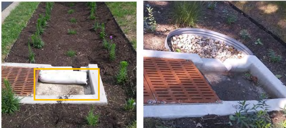
Figure 5. Bioretention cell with sandbag blocking the inlet and the same cell after sandbag was removed and runoff from street was routed into the practice. Blocking of the inlet structures preventing high-intensity runoff events from entering the practice immediately following planting to allow juvenile plants to become established in the bioretention media.
