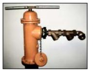
**5)** Carefully connect the two single check device assembly to the fire hydrant and have a permit holding technician present at ALL TIMES while the connection is in place.
