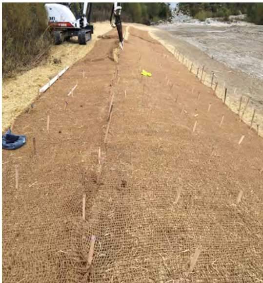
Figure 14. Revegetation Example During and After Construction
