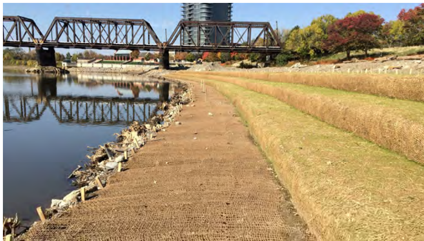
Figure 16. Reinforced Bank Example Under Construction
