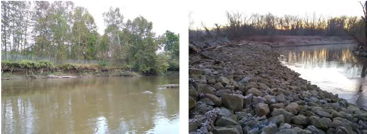
Figure 17. Riprap Revetment Example Before and After Construction
