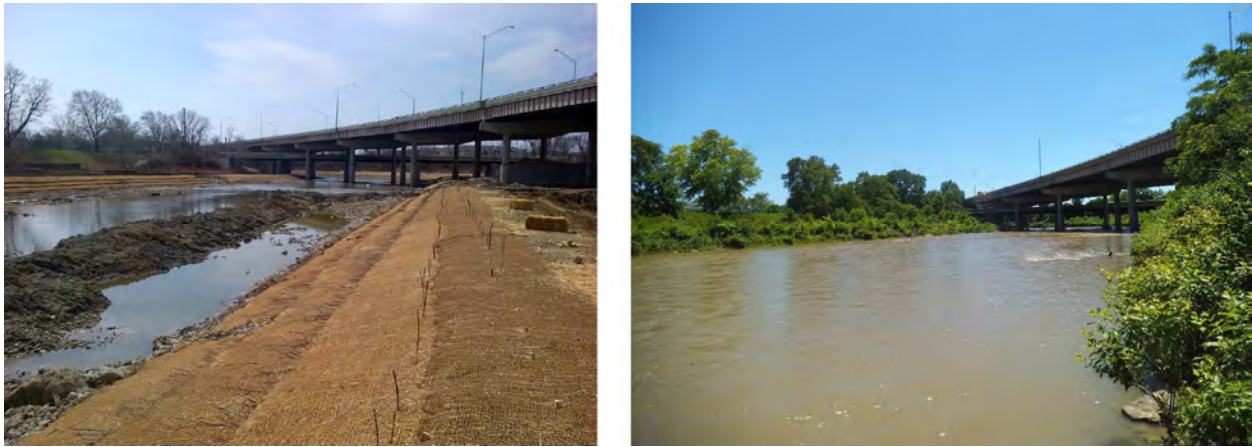
Figure 15. Bioengineered Bank During and After Construction
