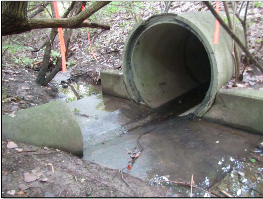
Photo 7: Inlet to existing 60 inch culvert routing tributary east under SR 315. I
