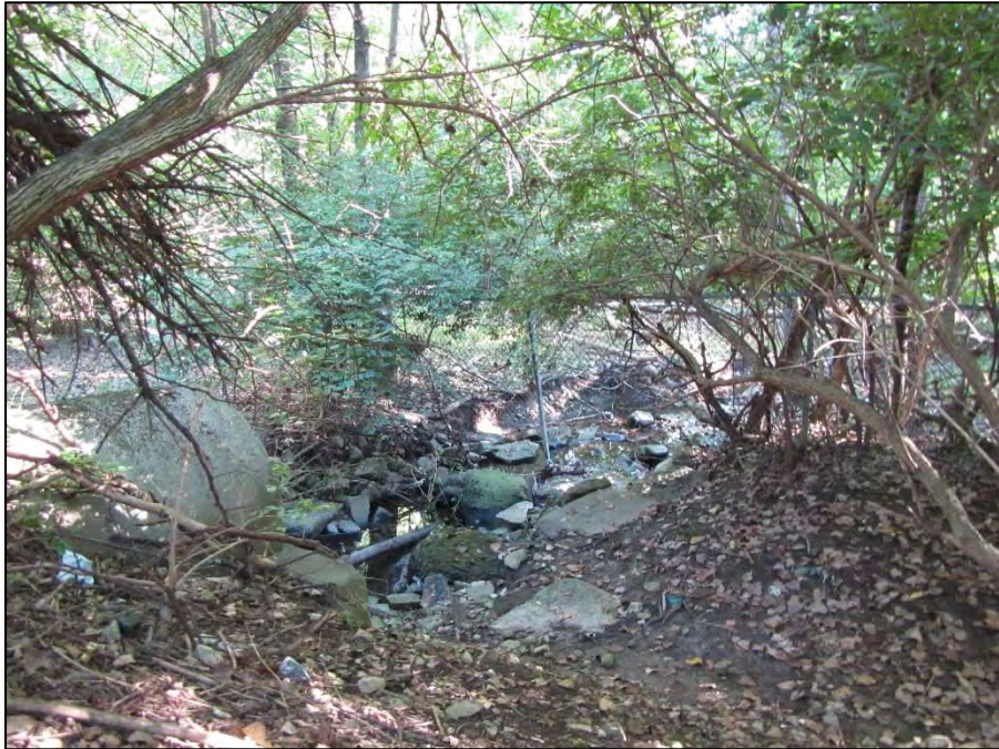
Photo 8: Looking downstream from 60-inch culvert outlet on east side of SR 315. From here, tributary flows to Olentangy River. Proposed new 60-inch storm culvert paralleling existing will also outfall to this location. Rock channel protection will be placed at outfalls.
