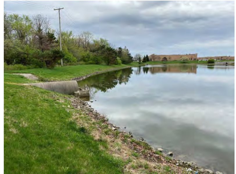
Photo 19: Representative view of the northwest stormwater basin that flows into Stream 9, located just west of the Site. Photo taken April 9-12, 2021.
