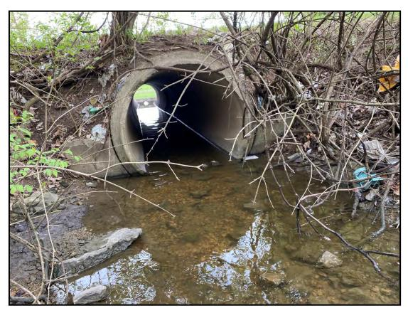
Photo 29 – Westerly view at the origination of Stream 9. This culvert pipe discharges surface water from a west adjoining storm water management pond.
