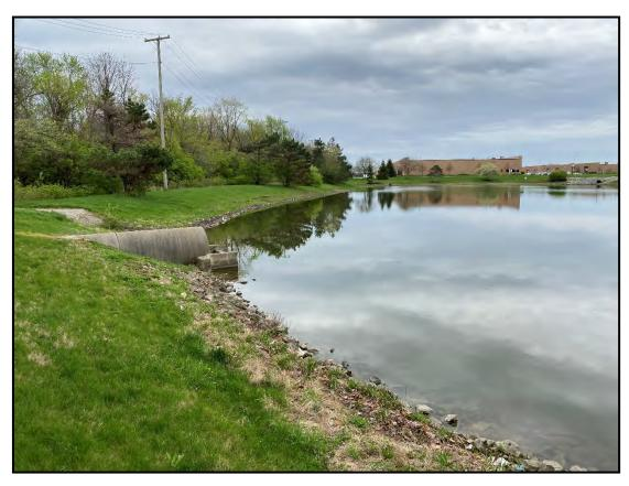
Photo 30 – Southwesterly view at the west adjoining storm water management pond directing surface water to Stream 9.
