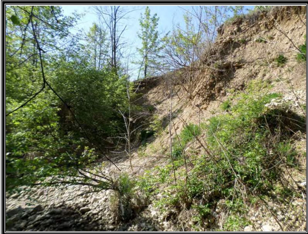
Photo 23 (4/20/16): Typical view of the steep sidewalls of the berm along the eastern side of the man-made drainage channel.
