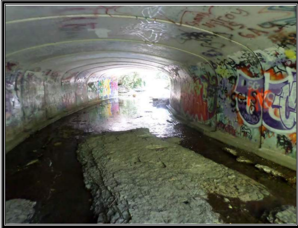
Photo 5 (6/14/16): Easterly view towards the site from the culvert beneath Dublin Road.
