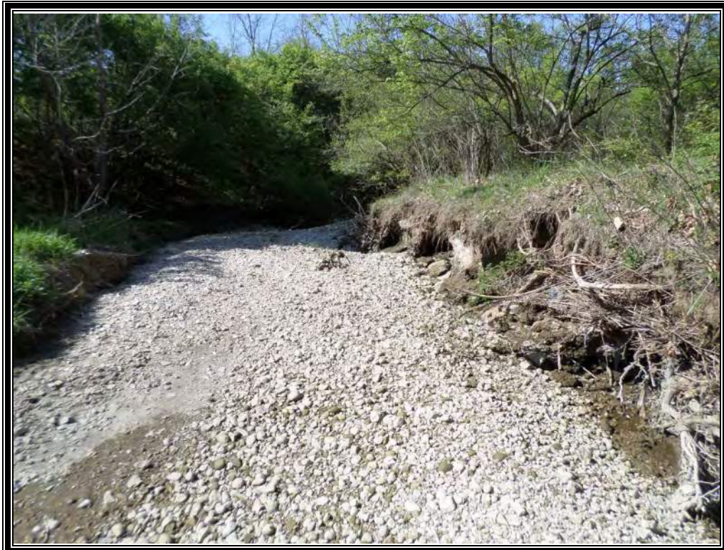
Photo 27 (4/20/16): Southwesterly view of the drainage channel on the south central portion of the property.
