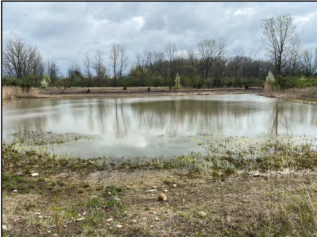
Photo 56 – Easterly view of Pond 2 on the South Section of the evaluation area.
