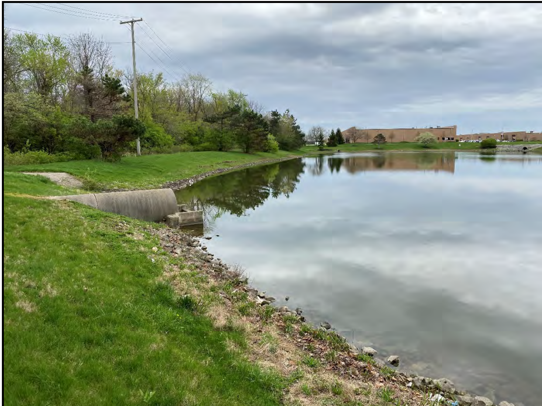
Photo 30 – Southwesterly view at the west adjoining storm water management pond directing surface water to Stream 9.
