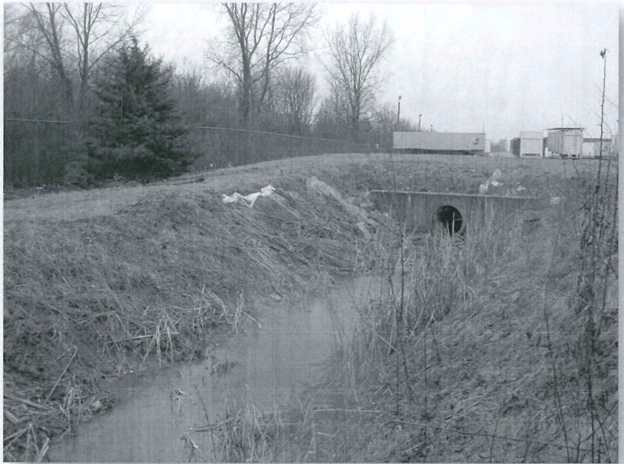
Plate 16. Overview of Improved Drainage Facing South
